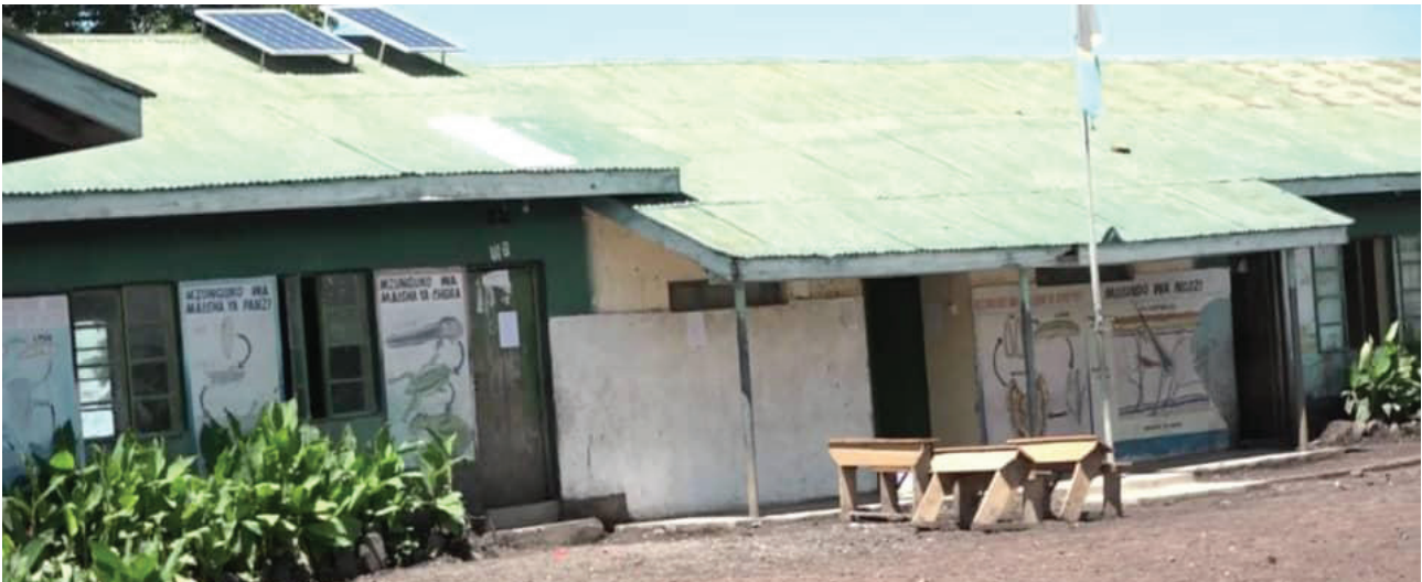
Photo No. 4.5: Endulen Boarding Primary School currently face shortage of pit latrines with 700 pupils forced to sleep four in a single bed. The school has two dormitories each with the capacity to accomodate 40 pupils.
