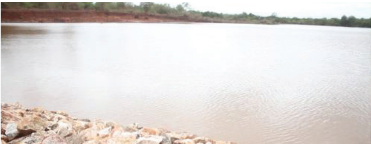
Photo No.3.2: Modern reservoir ( Cattle water pond) constructed at Msomera village
