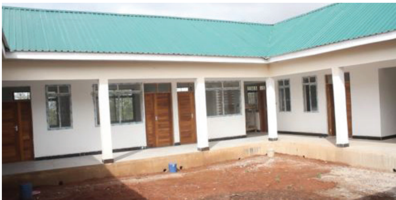
Photo No 3.3: A health centre under construction in Msomera village
