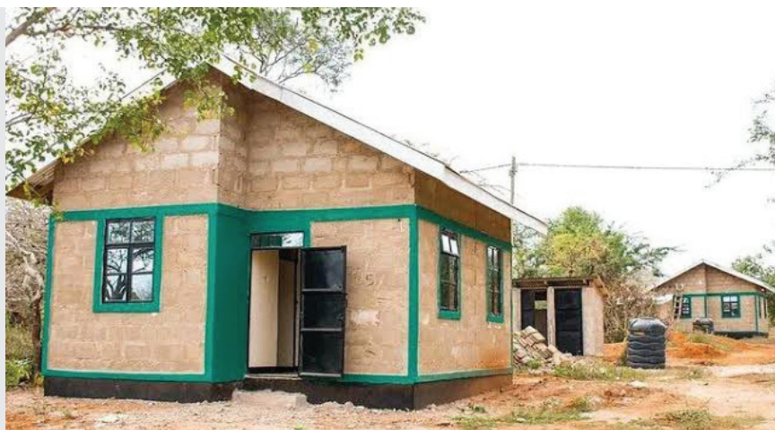
Photo No. 3.6: A model three-bedroom house built at Msomera village
